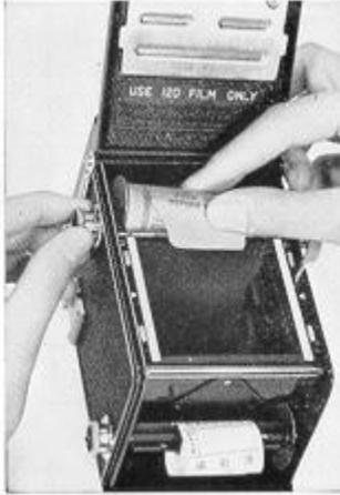
After taking all 12 pictures turn the Film Winding Knob about 6 turns, to take up the remaining film. Then open the camera and remove the film.
